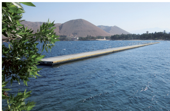
Floating breakwaters such as this, in Haql, northwest Saudi Arabia, are manufactured from reinforced concrete with an expanded polystyrene core. Ingemar manufactures modules of many sizes, including the giant of the family at 20 x 10m (66 x 33ft), 2.5m (8ft) high and weighing 185 tonnes apiece.
