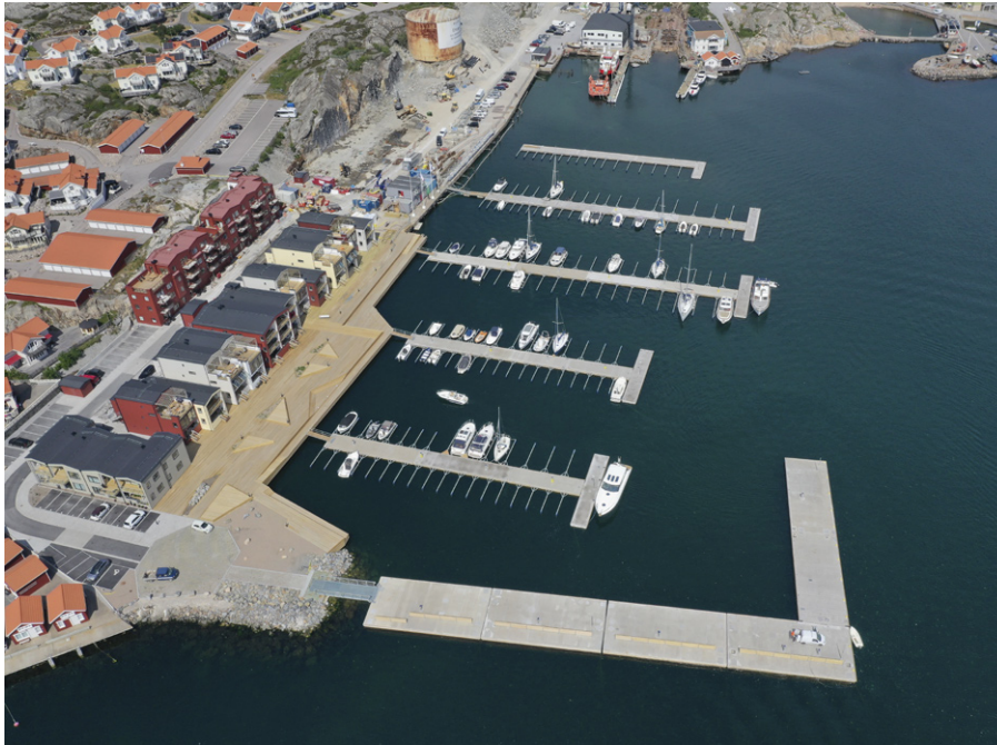
SWEDEN: Now complete and fully approved, the new floating marina built by SF Marina in Skärhamn on the west coast is a highlight in the mixed-use Kajen (Wharf) project. Supersizing was part of the design as the pontoons are twice as wide as normal and the SF floating concrete breakwater is by far the widest in the country.
