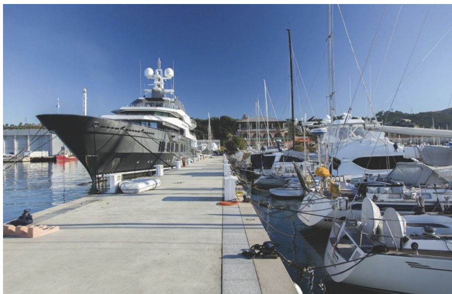
In 2016, Porto Lotti in the Gulf of La Spezia in northern Italy further boosted its megayacht berths with a custom-designed floating breakwater superyacht pier.
